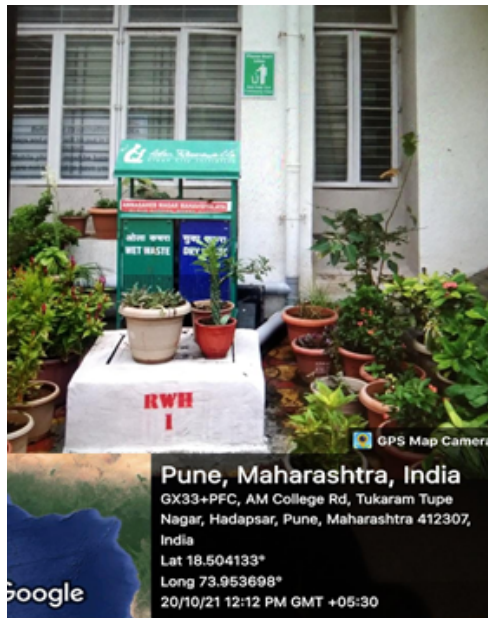
Rain harvesting unit 1
